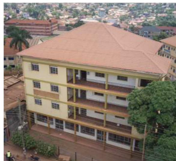
Ongoing construction of the Campus main building
