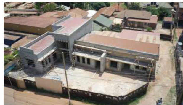
Ongoing construction of the ECUREI Research & A.I Center
